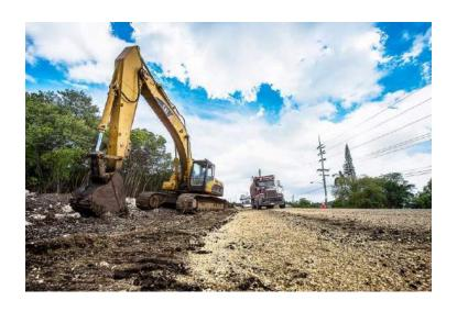
The National Roads Authority's (NRA) widening project is expected to provide an increase in vehicle capacity and reduction in traffic congestion during the peak hours of the morning and evening. NRA workers are widening the sub-base of the road, mainly the section from the Silver Oaks Roundabout to Halifax Drive on the south side of the roadway for about a mile.
